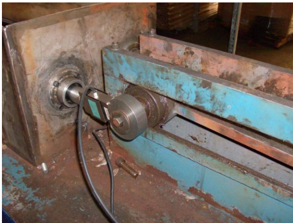
Figure 3 - Installed Load Cells
